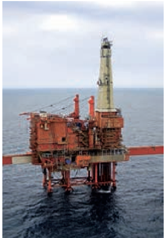
Boreplattformen Valhall DP. Foto: BP Norge AS
