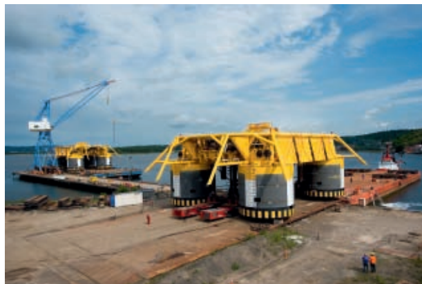
Constructing templates for Ormen Lange.
