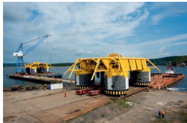
Constructing templates for Ormen Lange.
