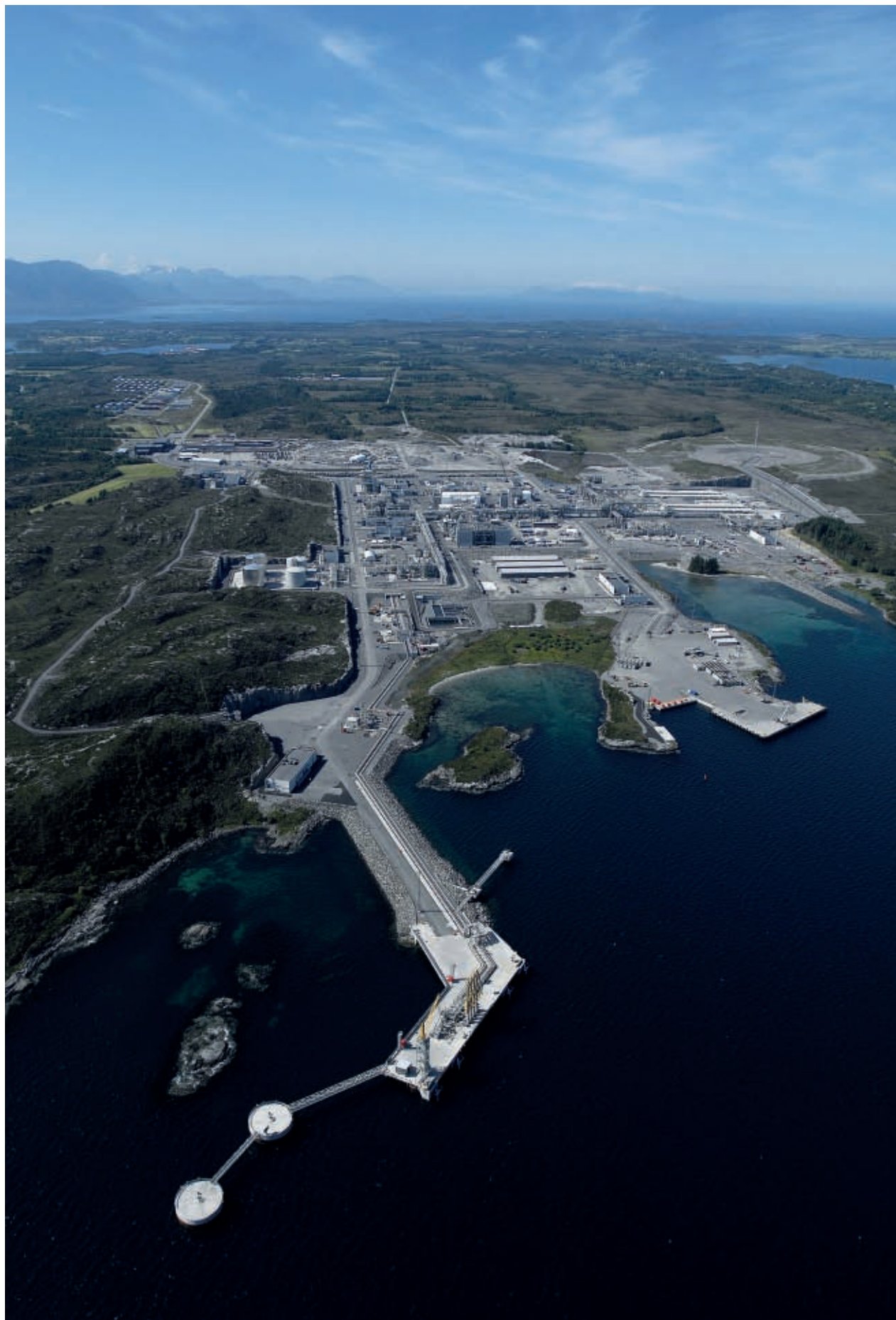
The Ormen Lange processing plant at Nyhamna, photographed in 2005. Photo: Øyvind Leren/Norske Shell
