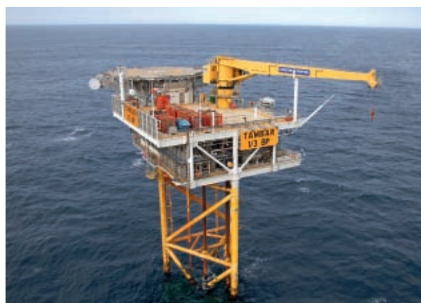
The Tambar platform. Photo: BP Norge
