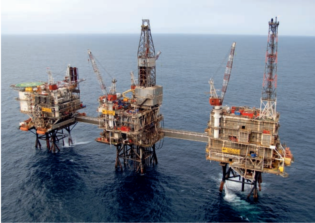
The Ula field. From left: the QP quarters, DP drilling and PP processing platforms. Photo: BP Norge
