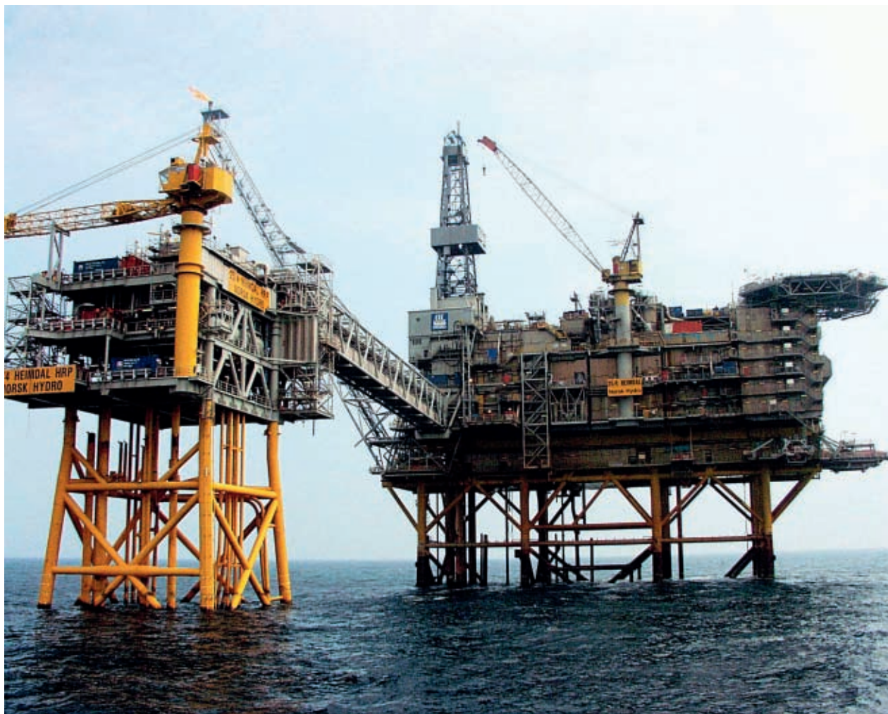
The Heimdal platform, with the riser installation in the foreground. Photo: Kjell Andersen/Statoil
