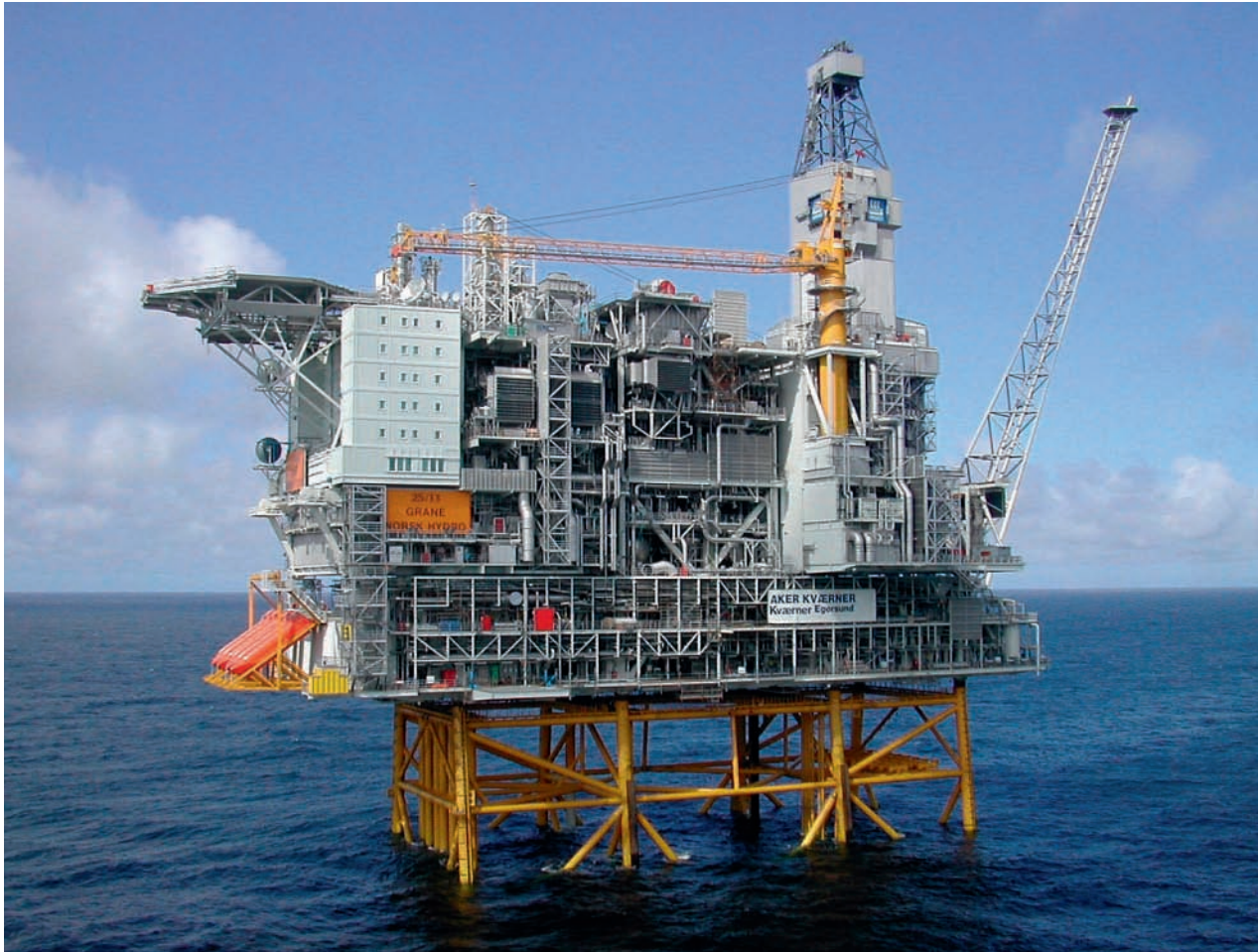
The Grane platform stands on a steel jacket. Photo: Norsk Hydro
