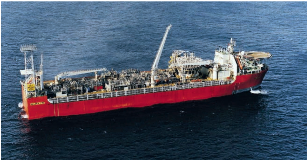
The Balder FPSO. Photo: ExxonMobil
