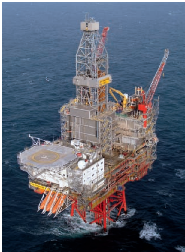
The Ringhorne platform. Photo: ExxonMobil
