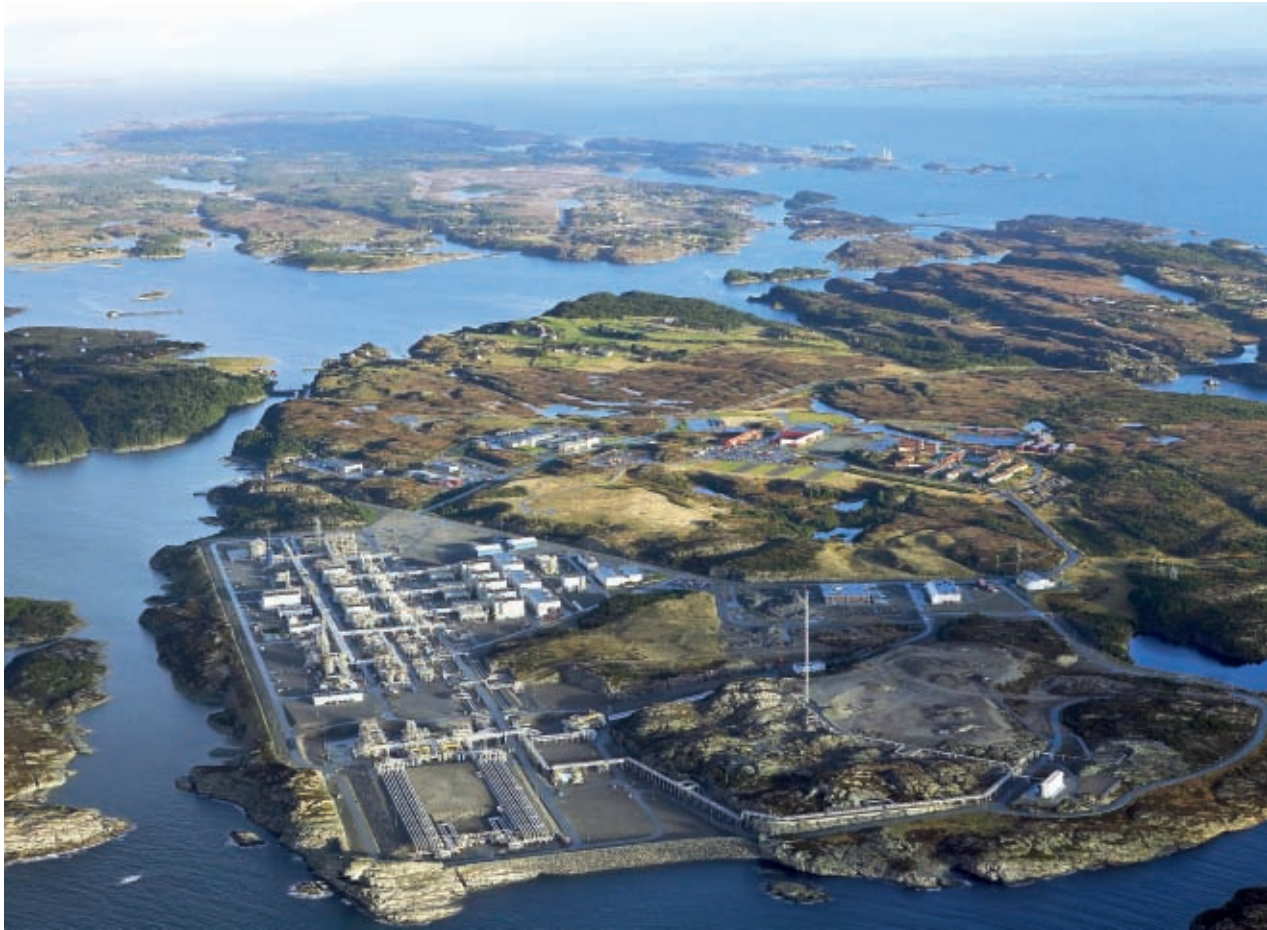
The Kollsnes processing plant. Photo: Dag Myrestrand/Statoil
