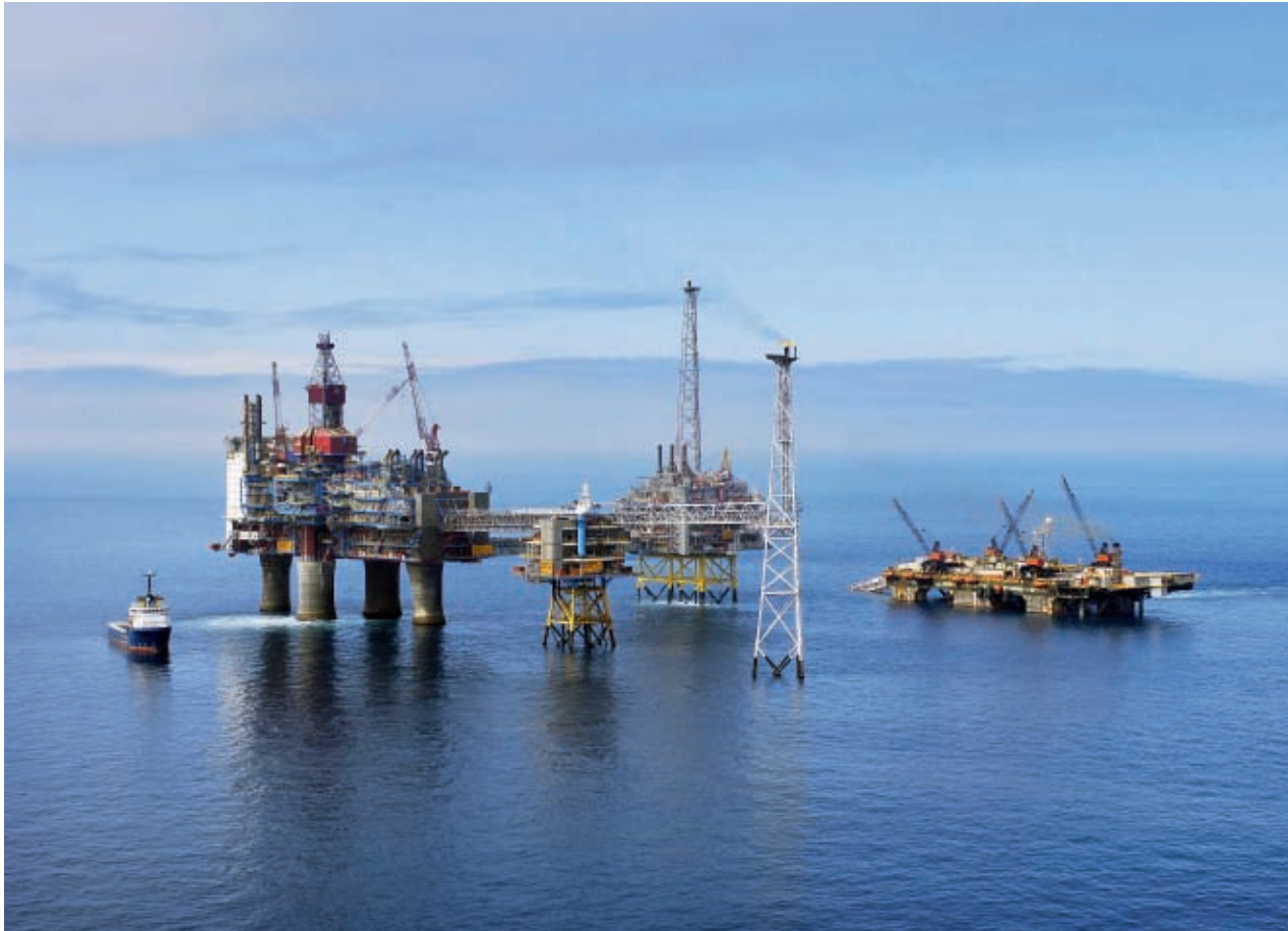
Laying Langed during 2005. From left: Sleipner A, R, T and the flare stack. Pipelay barge Acergy Piper is on the right. Photo: Kim Laland/Statoil
